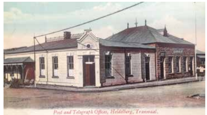
Post and Telegraph Office, Heidelberg, Transvaal.
