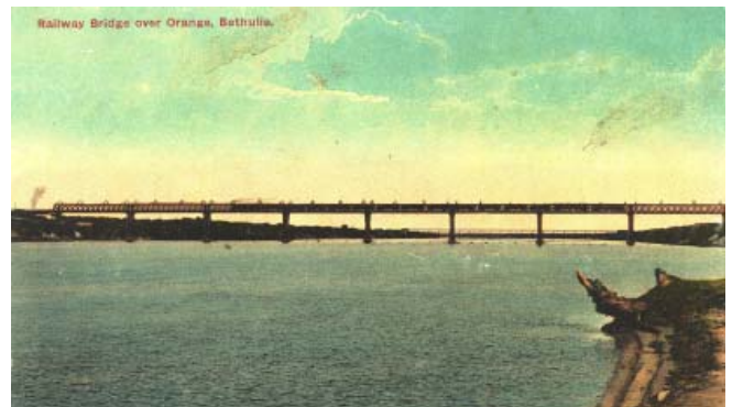
Figure 3. Bridge over the Orange at Bethulie, OVS.
